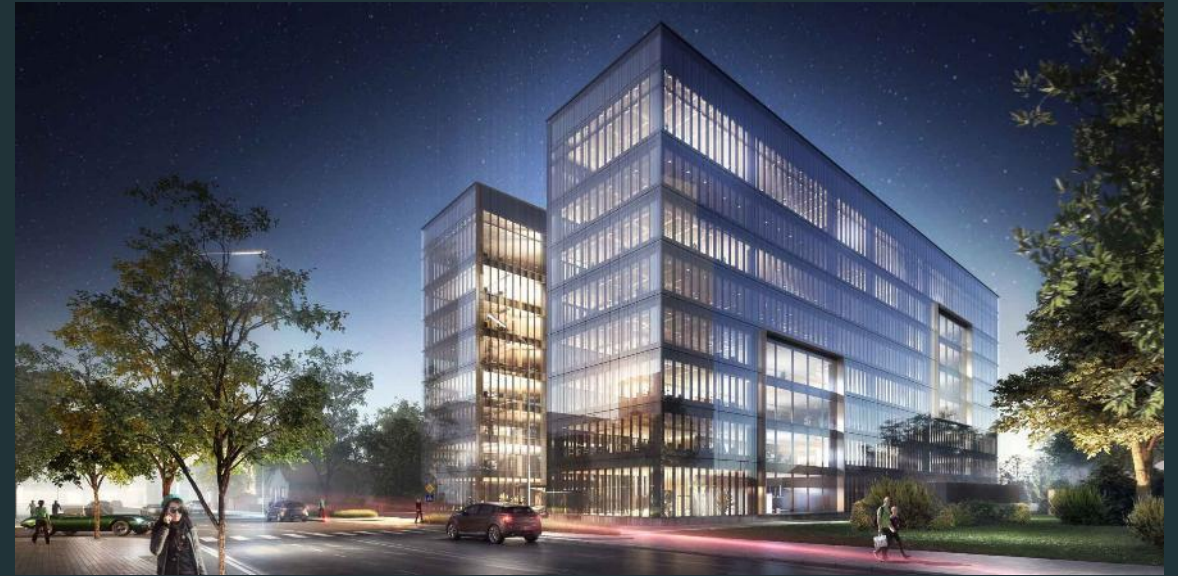
Lvivo 37, Vilnius BREEAM New Construction Outstanding
